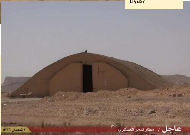
A hardened shelter with doors at Tadmur (Palmyra) airbase in central Syria. Source: https://www.bellingcat.com/news/2015/05/21/islamic-state-captures-tadmur-palmyra-in-new-sudden-streak-of-offensives/
