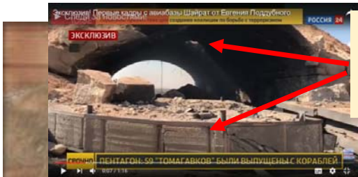
Pair HAS with roof penetrated by missile and debris outside
